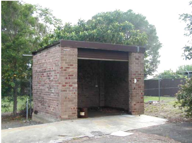
Figure 22. The Flammable Goods Store
