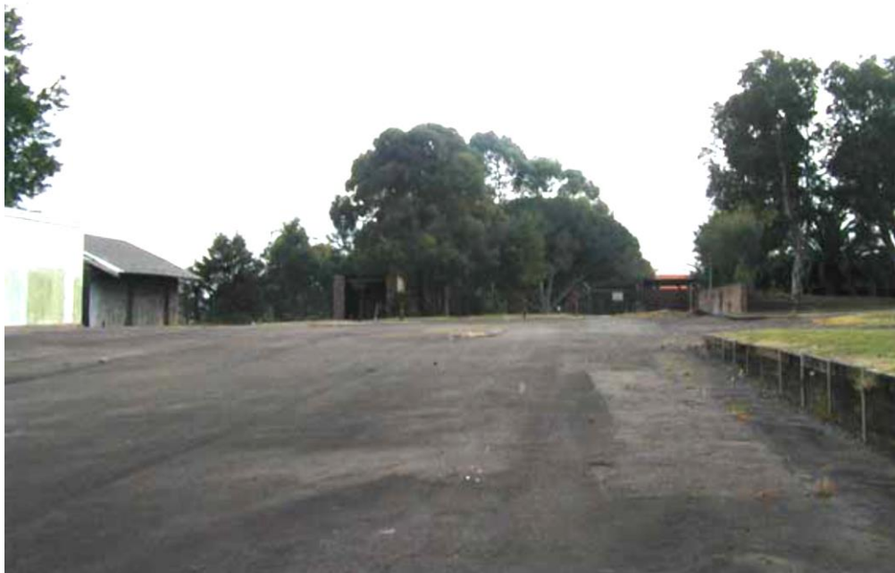
Figure 23. Asphalt-paved car parking area on the western side of the reservoir
