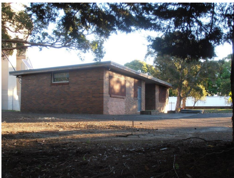
Figure 21. Depot Office and Amenities Building
