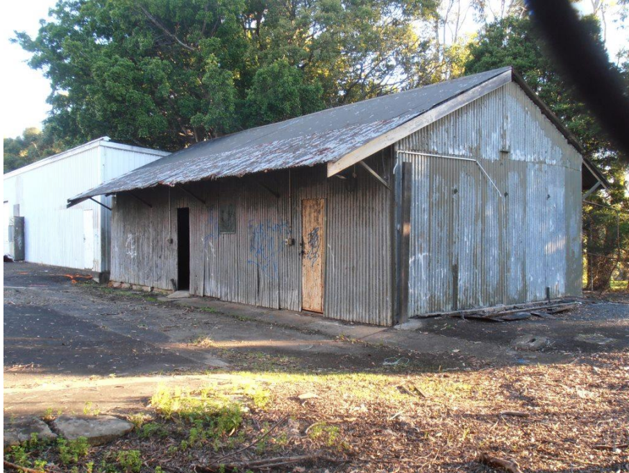
Figure 20. Corrugated iron shed
