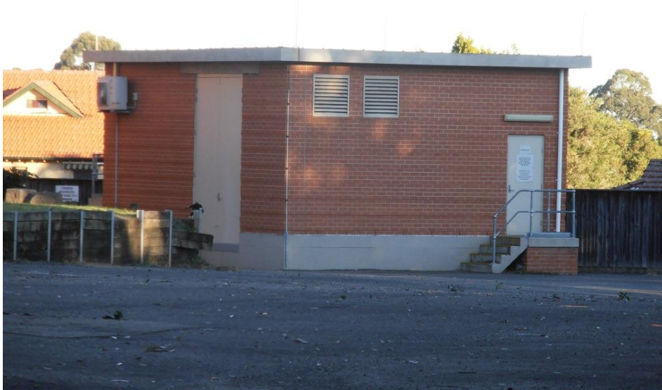
Figure 18. City Tunnel Ventilation and Secondary Access facility building
