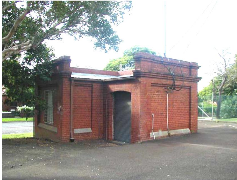
Figure 16. The Valve House for Ashfield Elevated Reservoir
