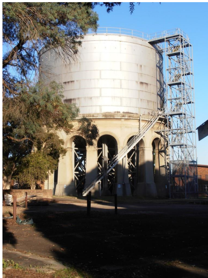
Figure 15. Ashfield Reservoir (Elevated) (WS 0003)
