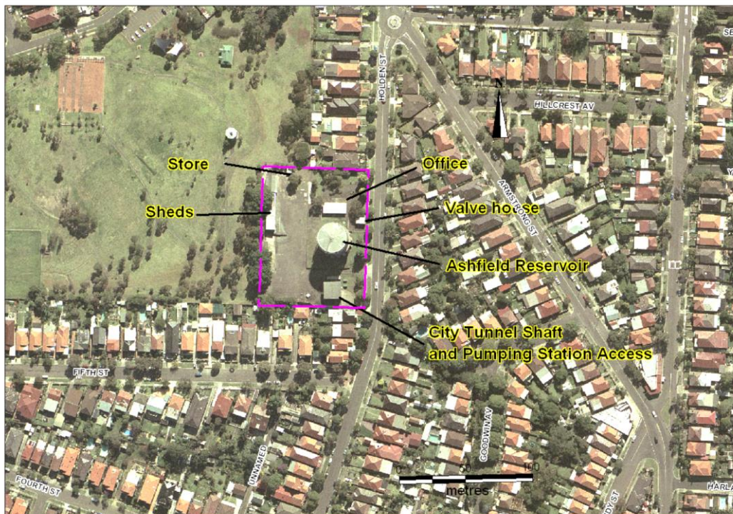
Figure 14. The Ashfield Reservoir site, showing the major components (CMP op cit)
