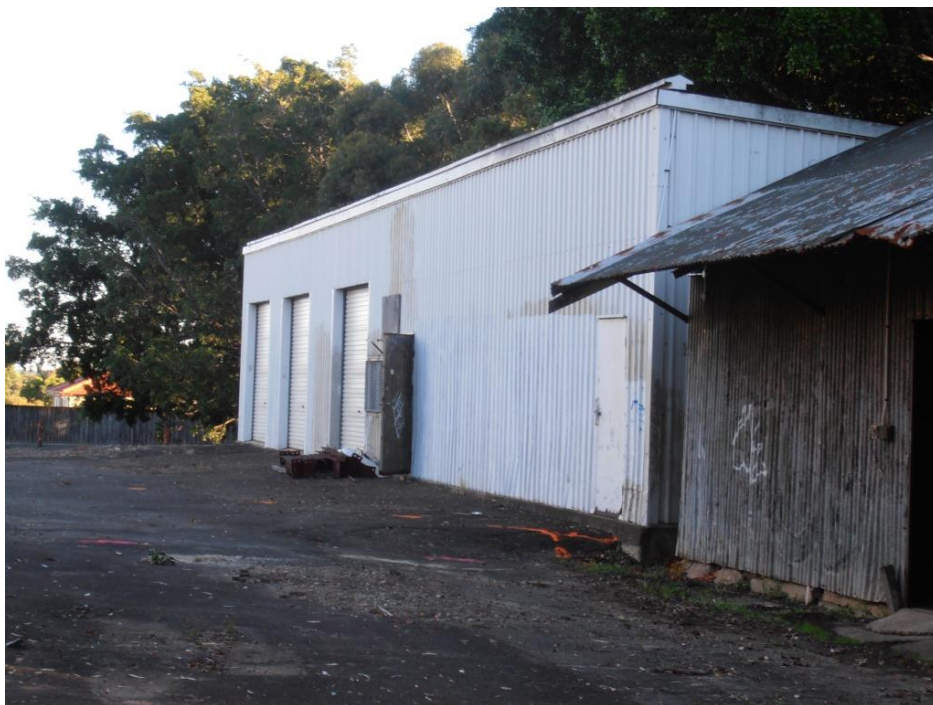
Figure 19. Sheet metal shed
