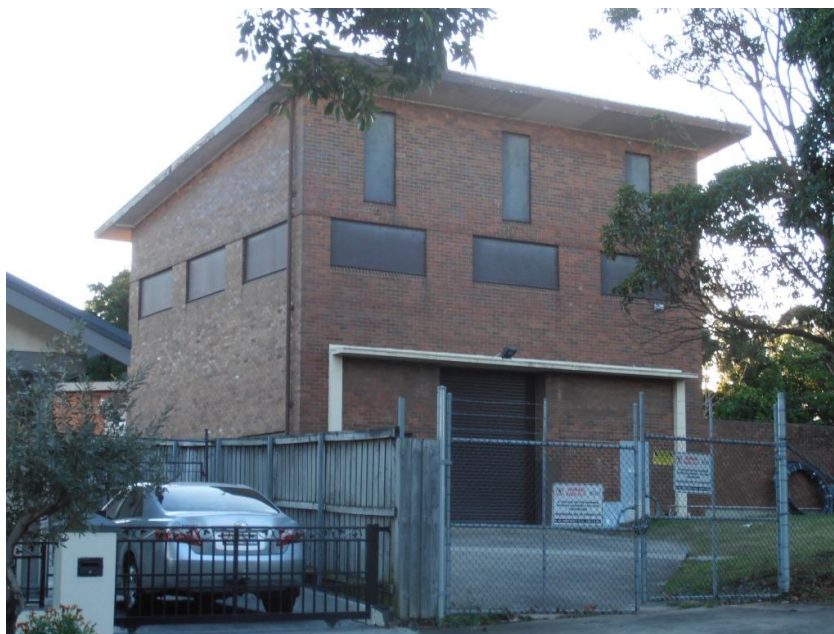
Figure 17. City Tunnel Access Shaft and Water Pumping Station building
