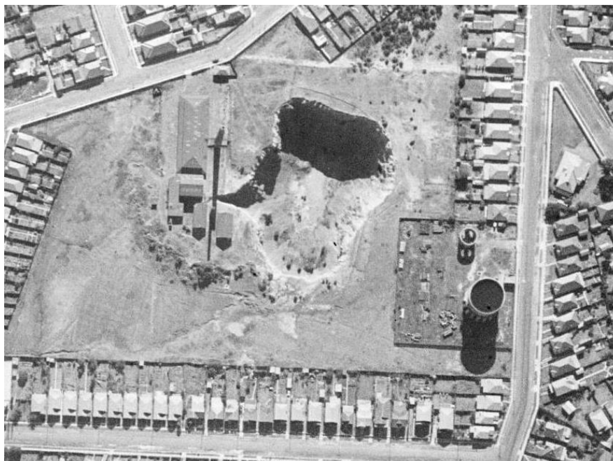
Figure 8. Ashfield reservoir site in 1943 - The brick stand for the original reservoir is visible on the north side of the 1914 reservoir and the land includes the second allotment to the west of the first. The third allotment, on the south side, has not yet been acquired. (Source: LPI Six)
