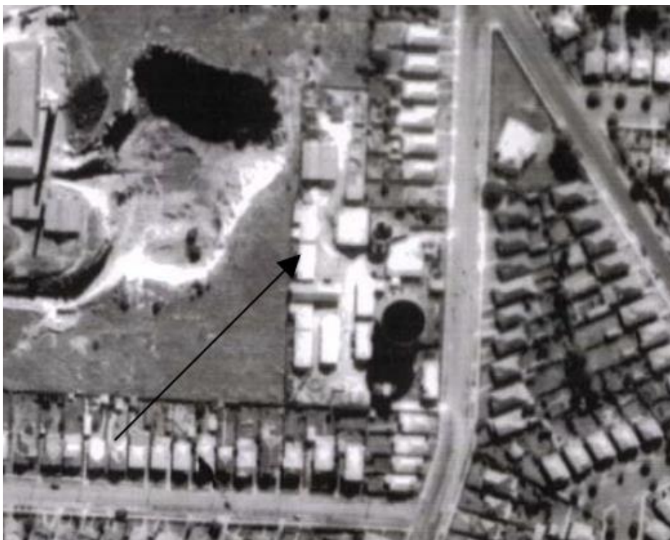
Figure 12. Aerial Photo of the site in 1951, showing the numerous buildings on the site associated with the construction of the City Tunnel. (Photo: Sydney (Cumberland) Run 14 May 1951 12" 12200)(Source: LPI)
